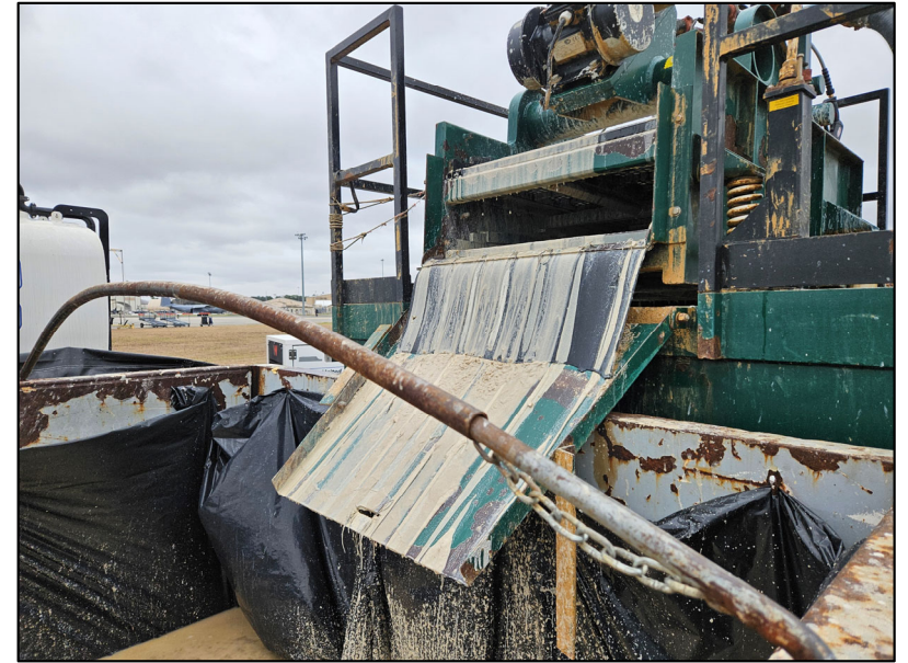
Drilling mud recycler
