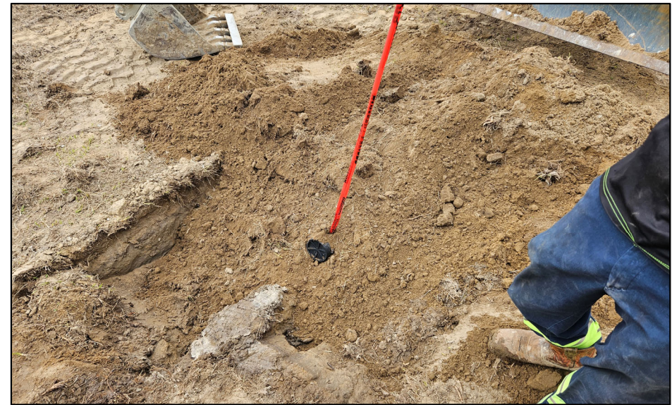
Well capped for temporary burial
