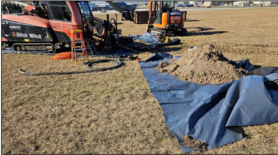
HDD drilling
