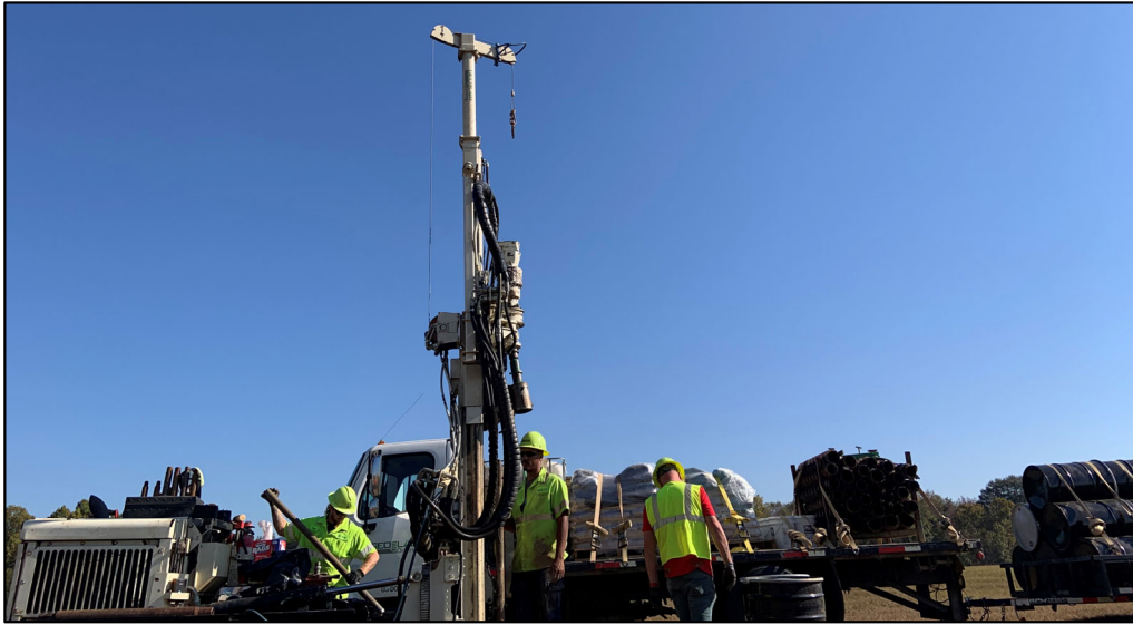
Vertical well drilling
