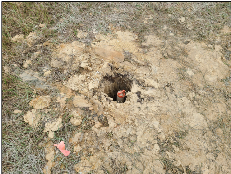
Vertical well ready for temporary burial
