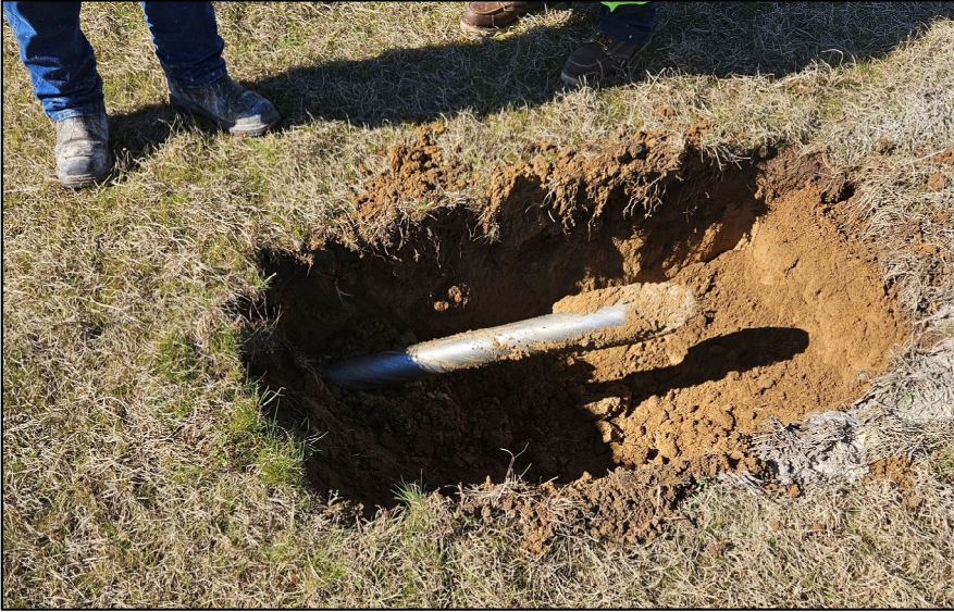
HDD exit pit
