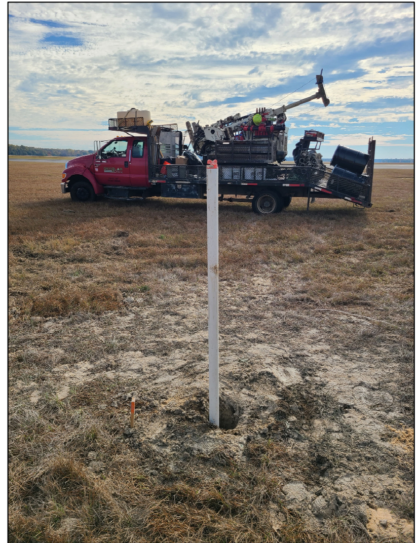
Installed vertical well
