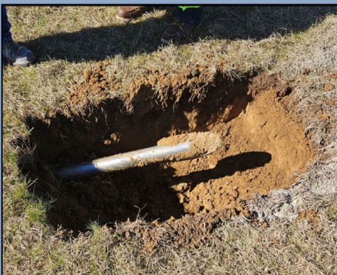
Photographs from installation of vertical and horizontal biosparge wells at SWMUs 59 and 60. Top left and right are vertical wells being installed. Bottom four are the horizontal drill rig, the drill bit, the drill bit at the exit pit, and the well casing being pulled back into the drilled hole.
