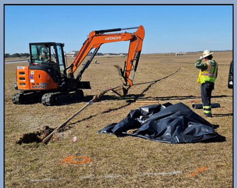
Photographs from installation of vertical and horizontal biosparge wells at SWMUs 59 and 60. Top left and right are vertical wells being installed. Bottom four are the horizontal drill rig, the drill bit, the drill bit at the exit pit, and the well casing being pulled back into the drilled hole.
