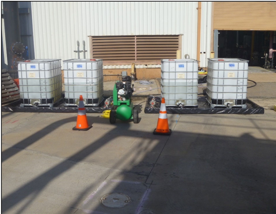
Ivey-Sol ® mixed in totes and injected with pneumatic pumps
