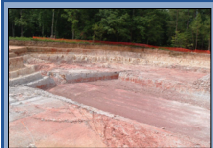
Kaolinitic Clay at SWMU 36 during Previous Excavation Activities
