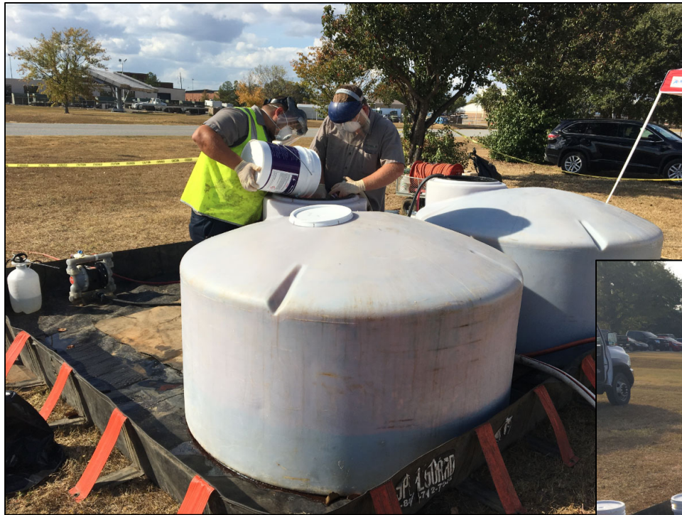
Addition of dry \text{KMnO}_4 to prepare 1.5% oxidant solution
