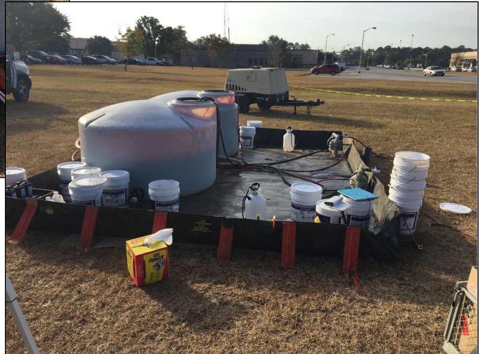
1.5% oxidant solution secondary containment during injection
