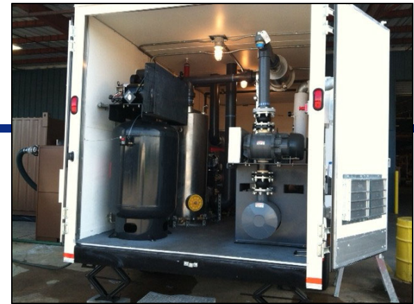
Remediation Trailer (↑) and LNAPL Collection Tank (↓)
