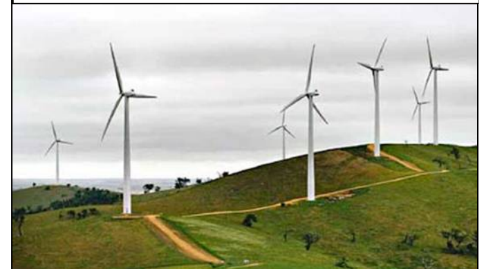
Wind Turbine Field
