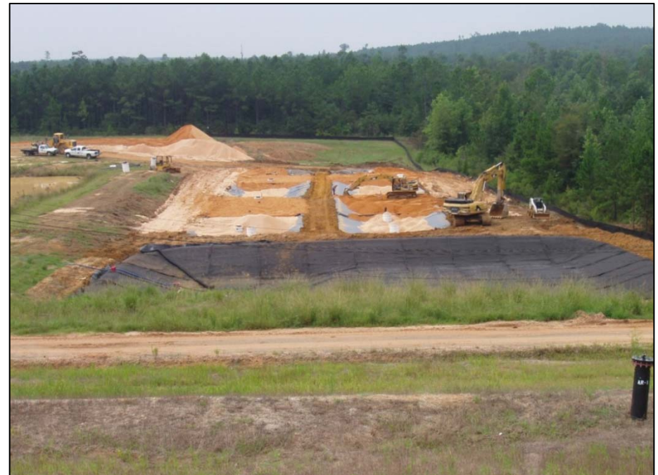
Wetland Construction - Placement of Pond Subsoil
