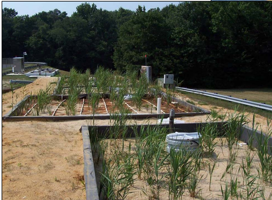
Pilot-Scale Wetland - Operational
