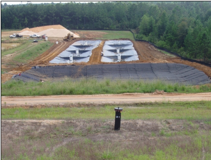
Wetland Construction - Liner Installation
