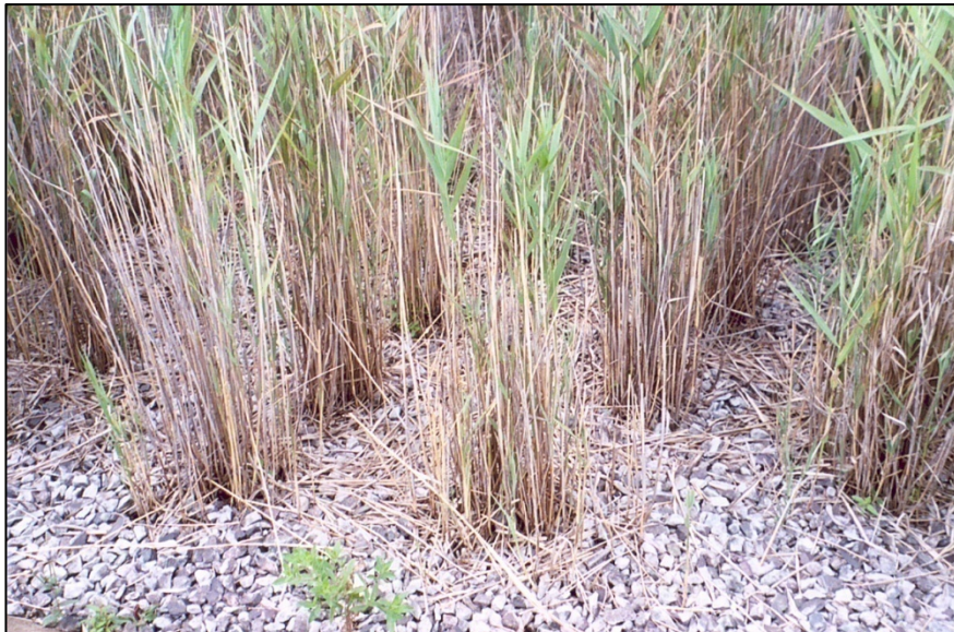
Plant Growth in Subsurface Flow Wetland
