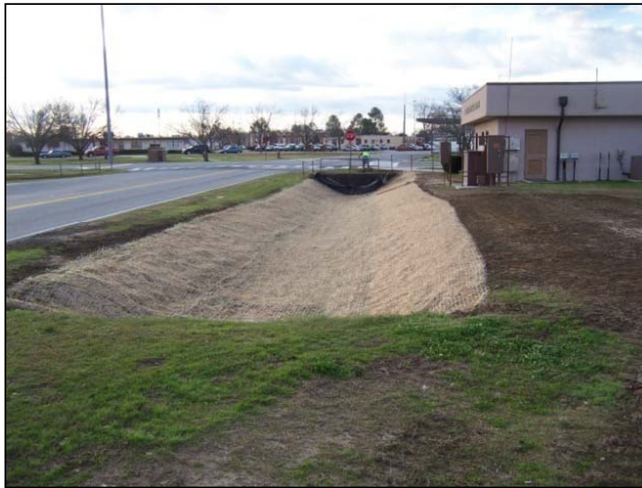
Erosion control matting
