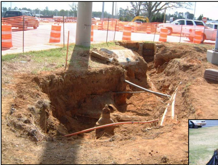
Exposing existing utilities
