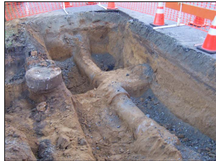
Exposing existing water pipe
