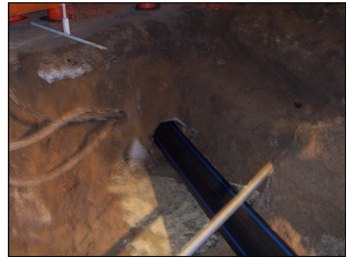
Installation of new of HDPE pipe
