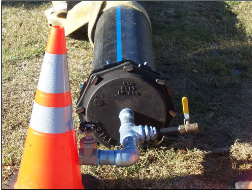
Valve assembly for disinfection of HDPE pipe
