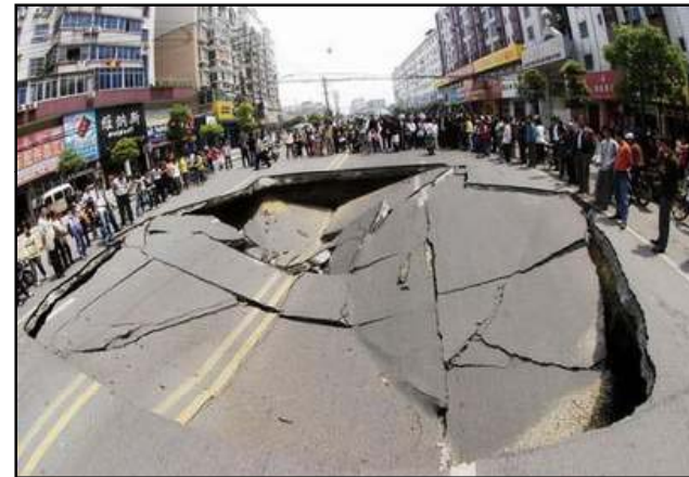
Public safety concerns
