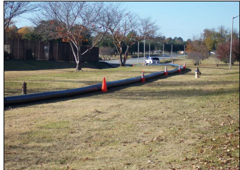
HDPE pipe fused on-site
