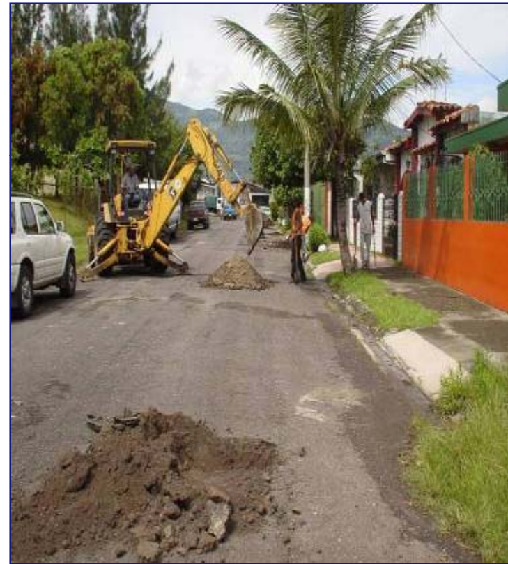
Typical excavation for pipe bursting
