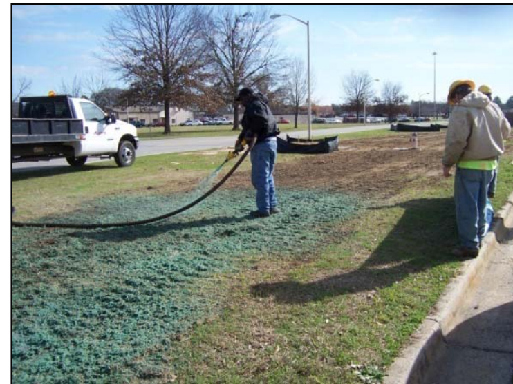
Hydro seeding disturbed area
