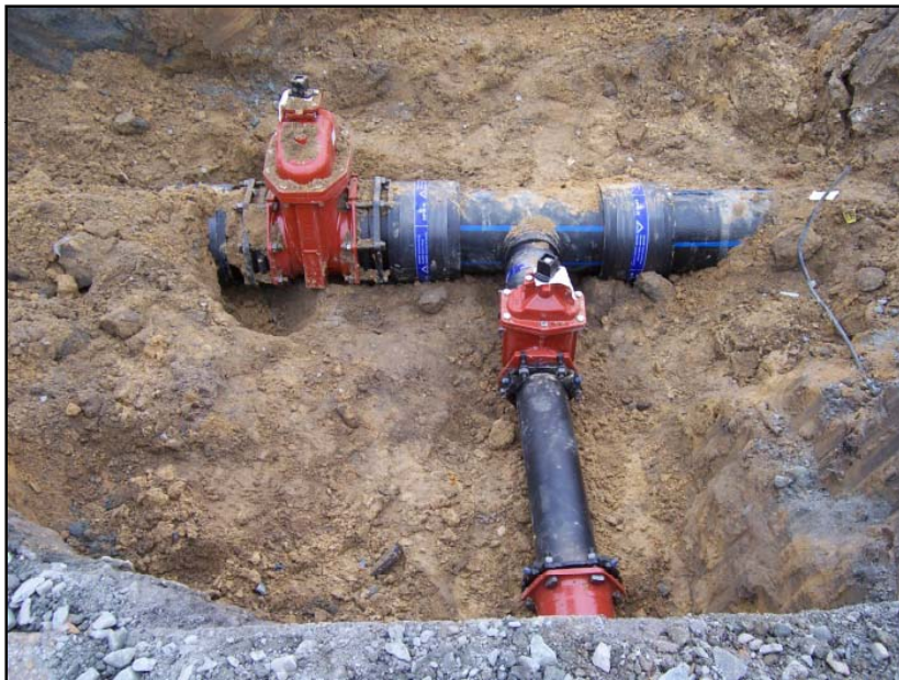
New pipe and valve installed
