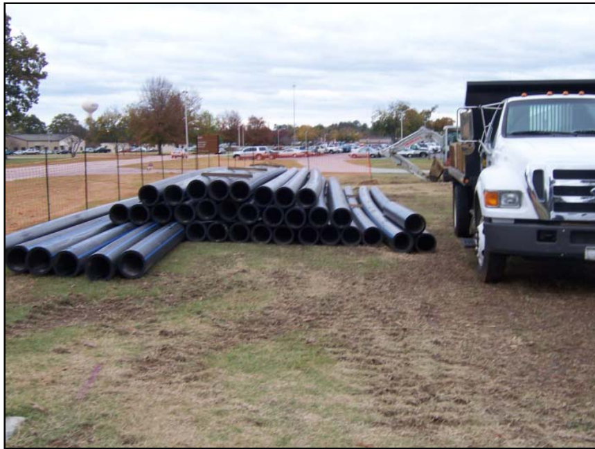
HDPE pipe storage on-site
