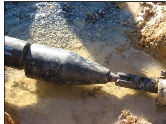
Expander head entering existing pipe
