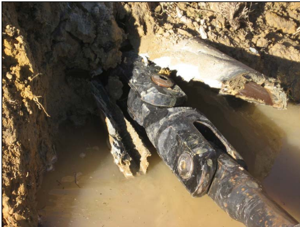
Splitter entering existing pipe
