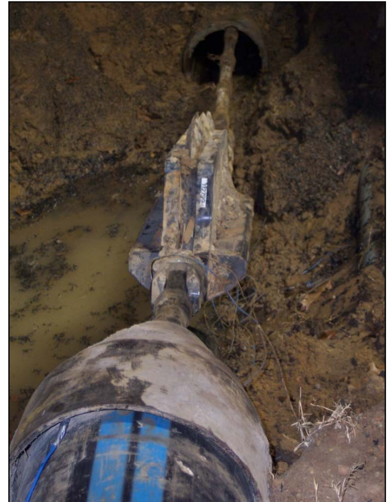
New HDPE pipe being pulled in place
