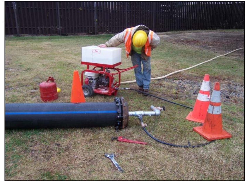
Injection of disinfection fluid into HDPE pipe
