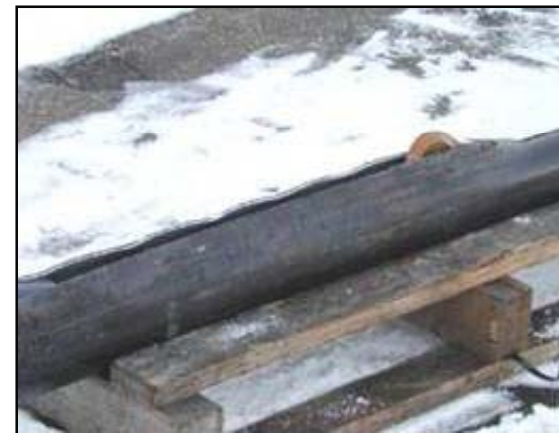
Cast iron pipe
