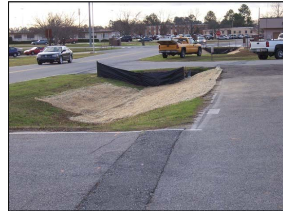
Access pit restoration
