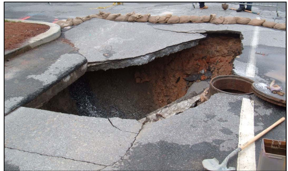
Sinkhole at Georgia Tech – 32 feet deep Caused by rainwater leaking into broken sewer pipe
