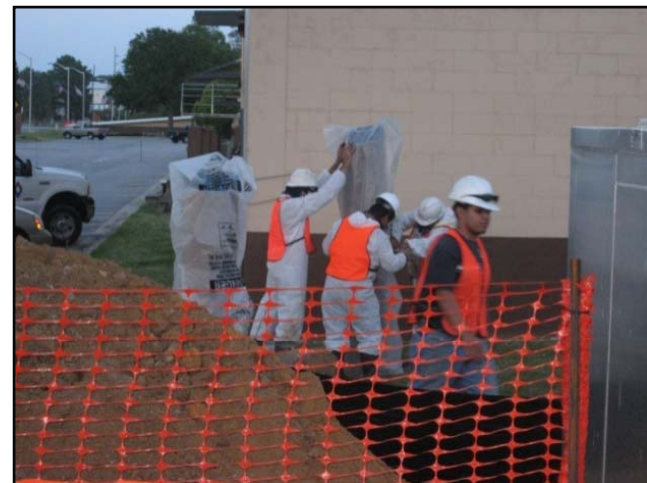
Removal of existing water main
