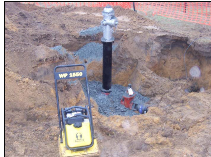
New fire hydrant installed
