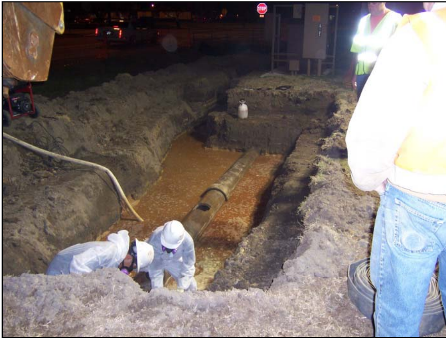
Removing existing pipe at access pit
