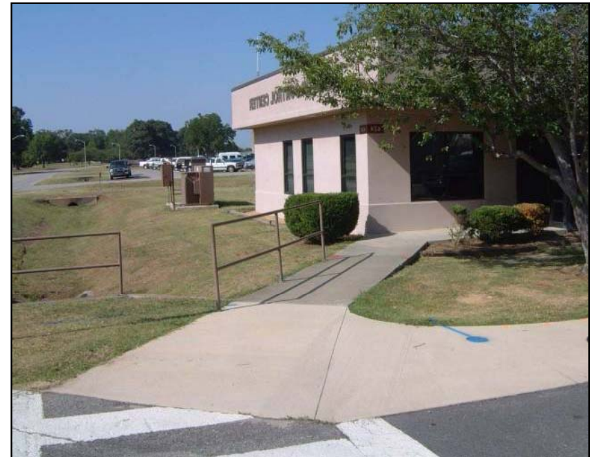
Page Road water main replacement site
