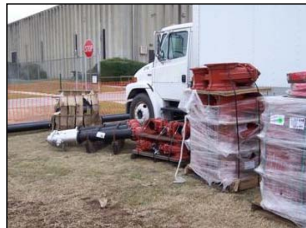
New valves and fire hydrants
