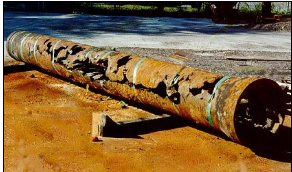
Deteriorated piping allows infiltration overwhelms collection systems and treatment plants
