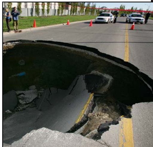
Sinkhole from leaking water line
