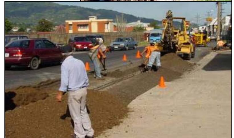
Traditional excavation to repair/replace utilities
