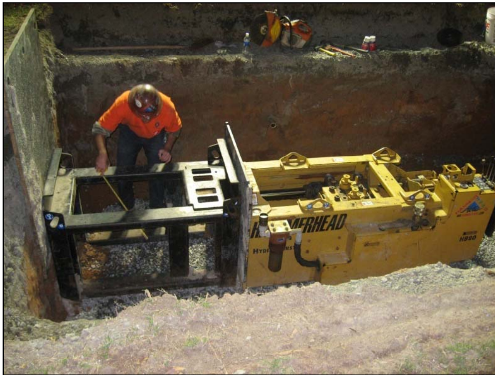
Pipe bursting pulling equipment
