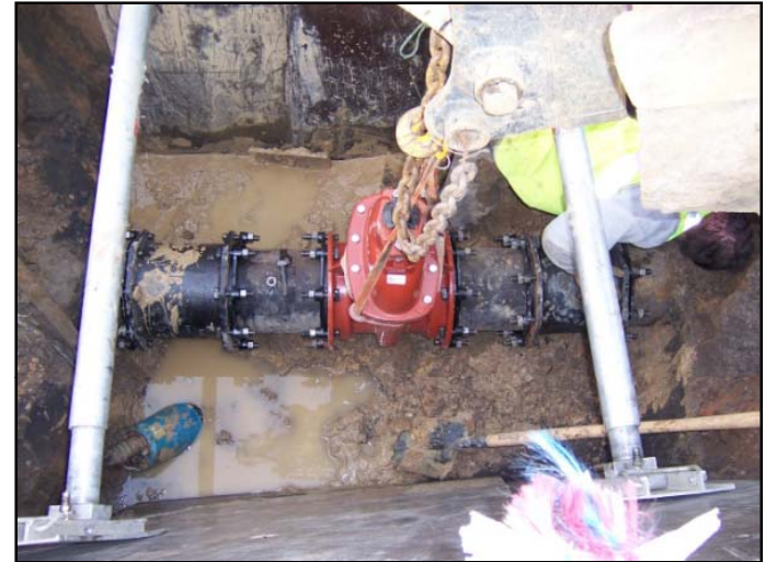
Lowering new valve in place
