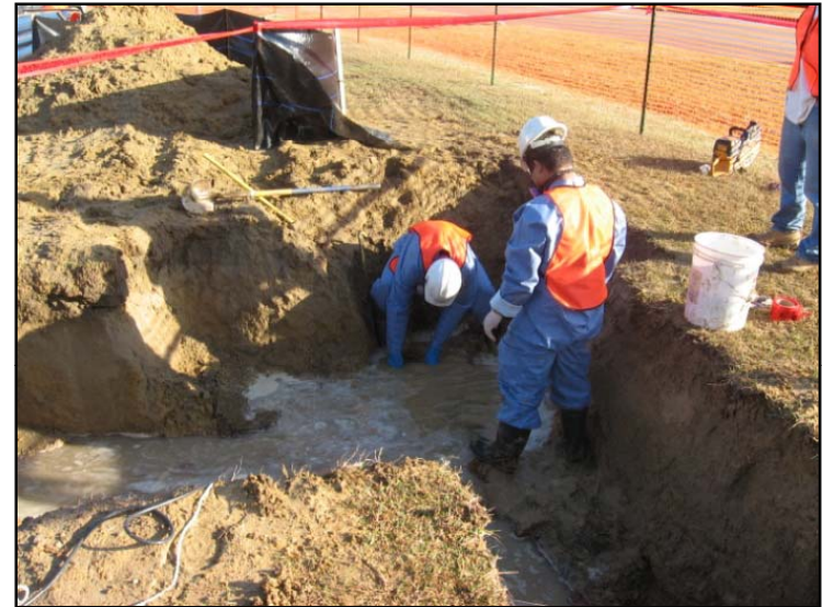
Pipe bursting access pit
