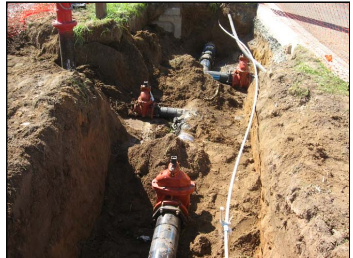
New valves installed
