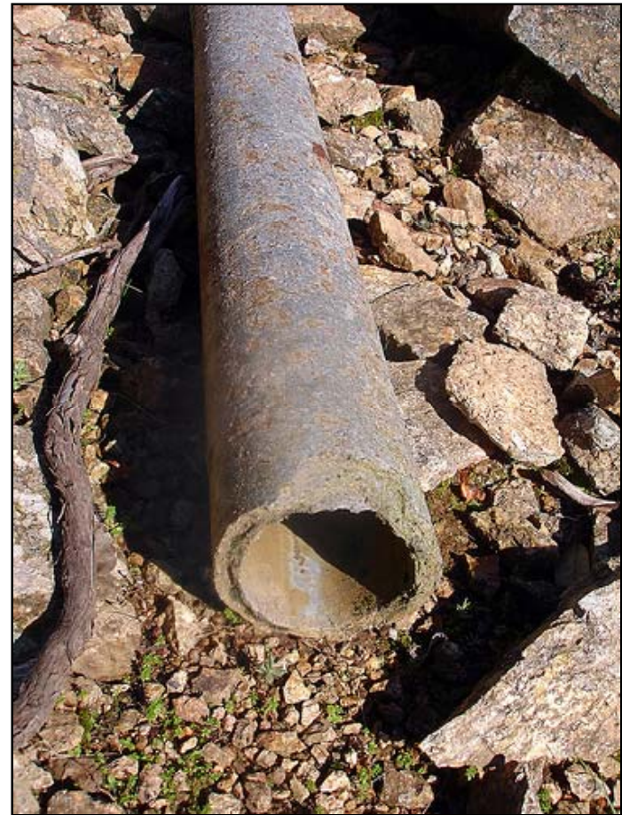
Asbestos cement piping
