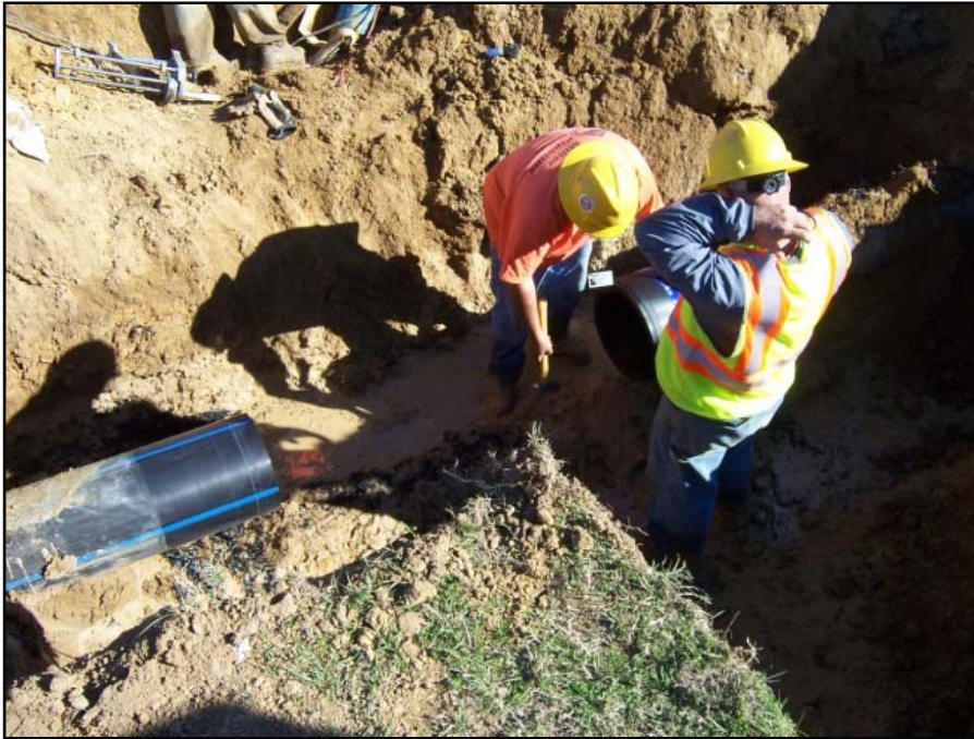
Installing new valve assembly
