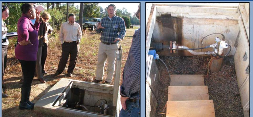
Mr. David Fortune explains the chemical dosing system at an extraction well vault (left). A close-up view of the extraction well head with the newly installed recirculation system to allow dosing of the deposit control chemicals (right).
