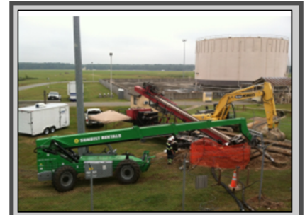
Installation of biosparge well.
