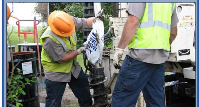
Placement of sand pack between well and augers.
