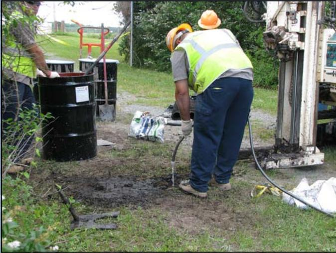
Drill crew hydrating the bentonite seal placed above the well screen with potable water.
