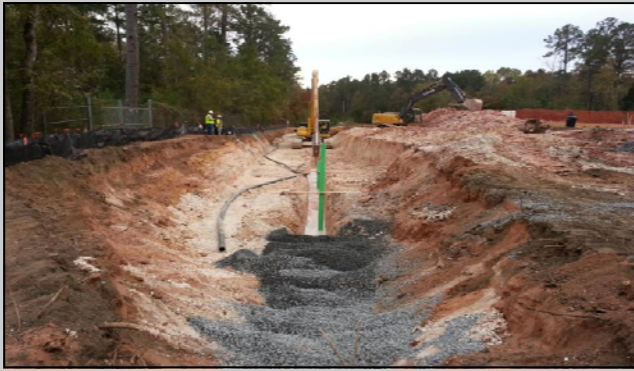
Excavation for the SVE Trench
