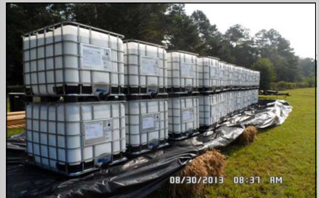
Staging Area with Secondary Containment for EOS Pro ®
