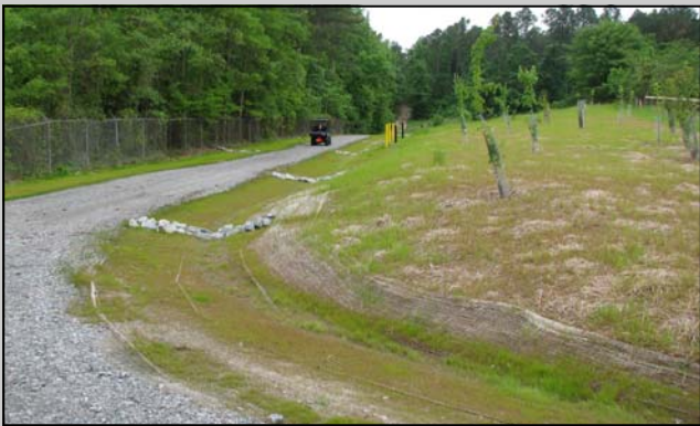
View Looking Down the Alignment of the AS/SVE Barrier
