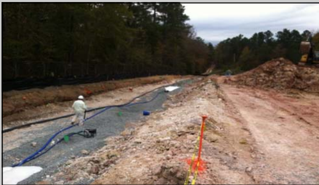
SVE Trench Backfilled with Gravel
