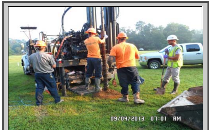
Installation of Typical ERD Injection Well
