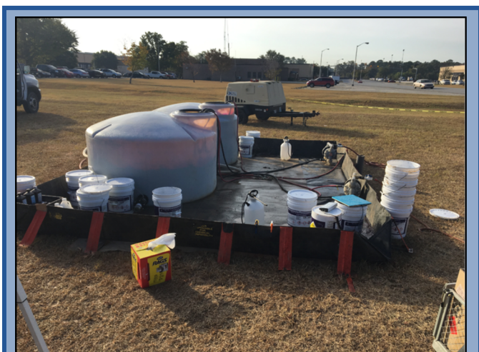
ISCO injections at SWMU 62.
