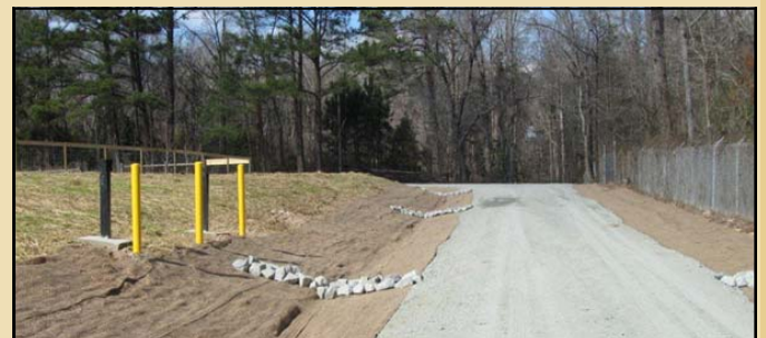
Perimeter Road after AS/SVE system construction
