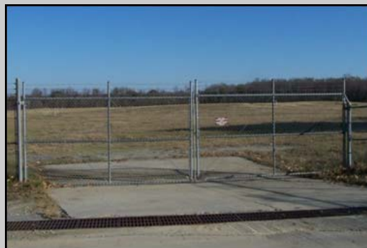
LF004 LUC (Fence and Locked Gate)
