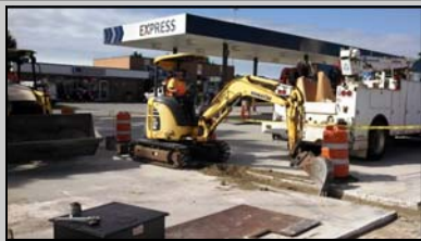
Trenching to Install Conveyance Lines for AS/SVE System
