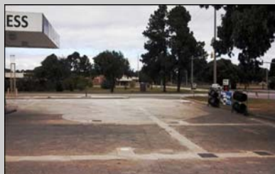
Area after Installation of Piping
