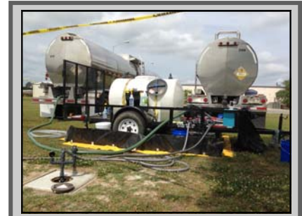
Tankers and Trailers for ISCO Injections
