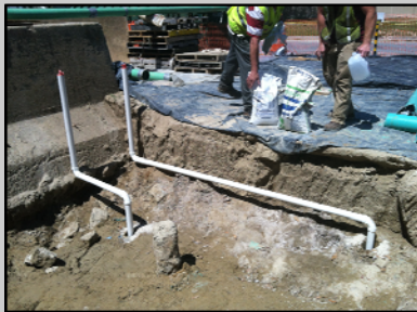
SVE Wells during Construction
