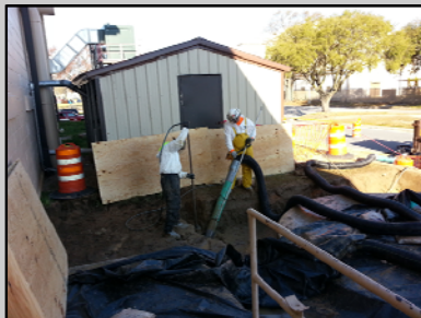
Hydrovac Excavation in Progress
