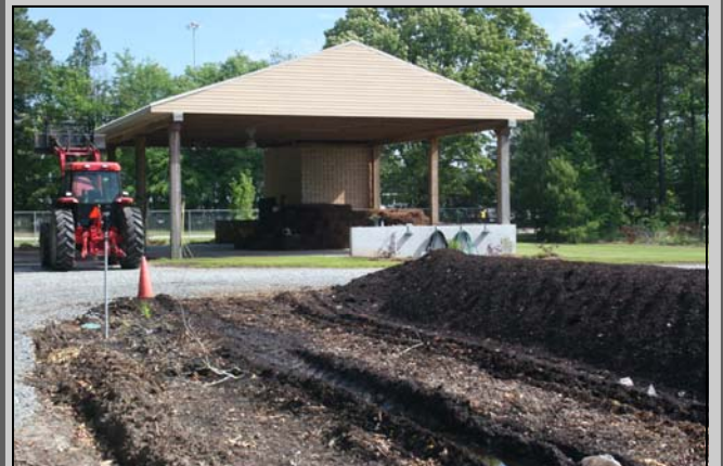
The composting facility recycles yard and stable waste for use in Robins AFB beautification projects.
