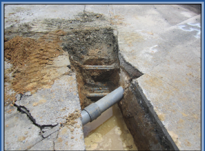
A large number of underground utilities were identified along the proposed alignment of one of the horizontal wells during a recent utility survey.
