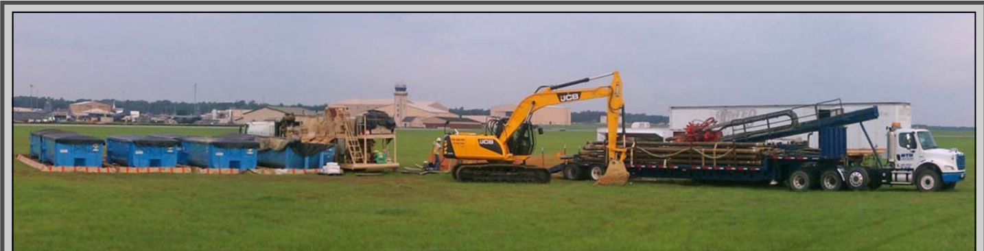
Drill rig set-up for HDD wells in flightline area.
