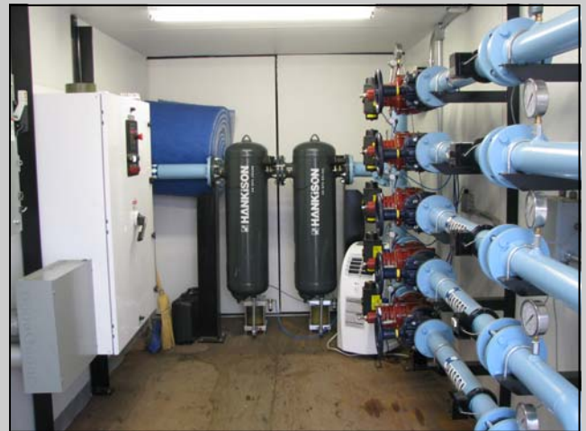
View inside the biosparge equipment compound. The manifolds for each of the five horizontal wells can be seen on the right of the photograph.
