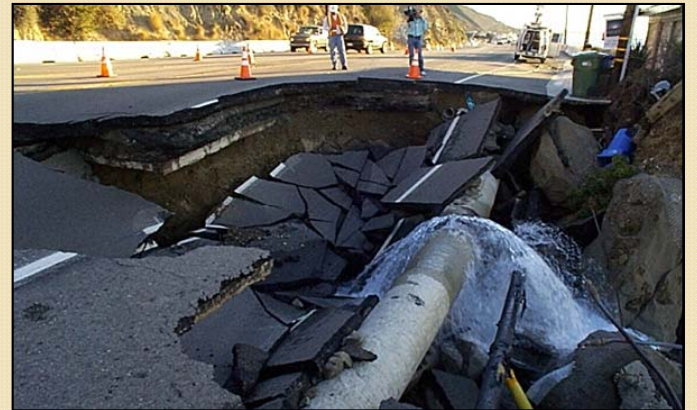
Aging infrastructure across the United States is causing problems with the drinking water infrastructure. Corroded pipes that collapse or break can result in sinkholes at the ground surface, interruption to service and traffic, and costly repairs.
