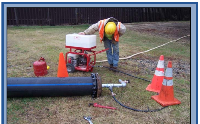
Prior to being installed, each section of pipe must be disinfected for 24 hours using a chlorine solution.
