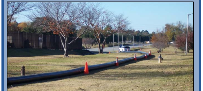
The entire length of pipe is laid out and welded together before installation.
