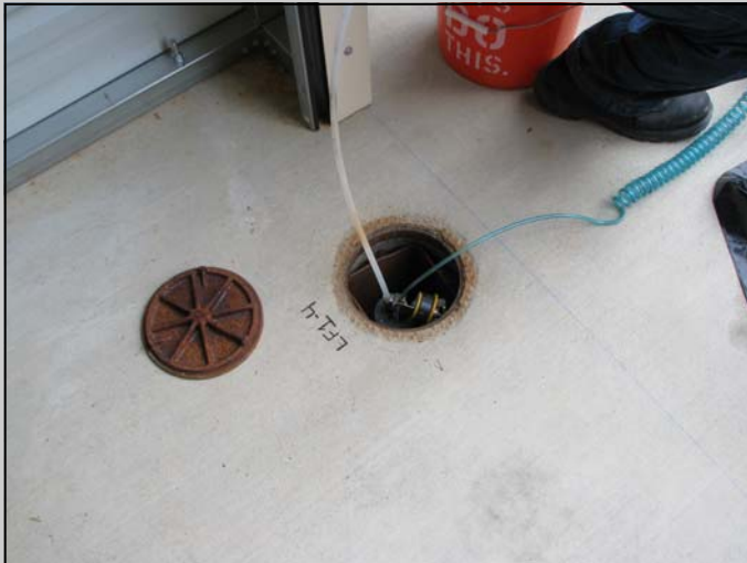
Close-up view of LF1-4 wellhead with bladder pump controls attached.
